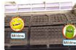
Thick dust on the air conditioner filter
